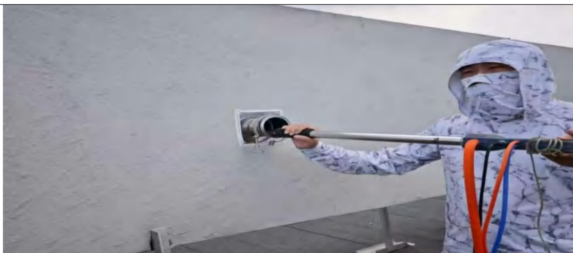
GLP 实验楼排气筒 1DA002
